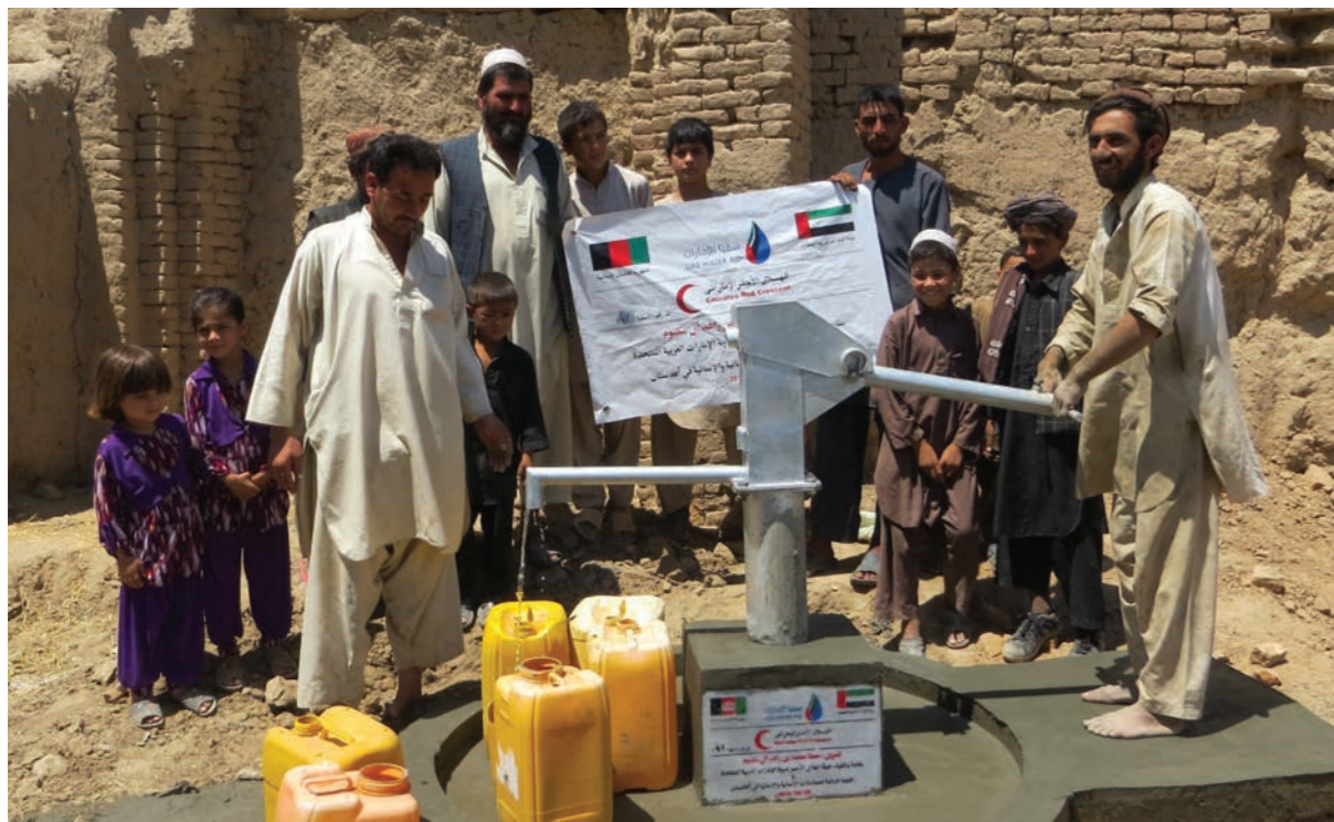
Drilling of wells in Afghanistan
